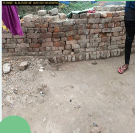
Fencing BR_BAHA CHAUKI_242931_015101_W1
