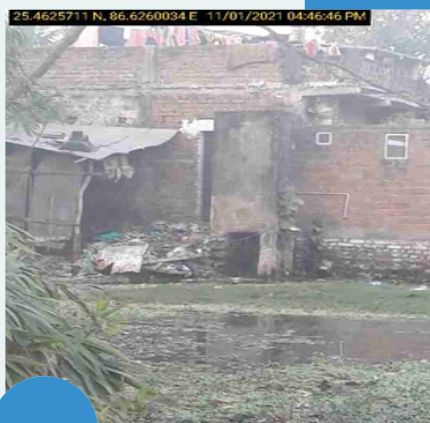
Wastewater Drainage BR_JHIKTIA_238718_014812_W2
