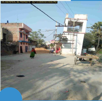
Construction site within 250 m BR_NAWADA_218378_014221_W1
