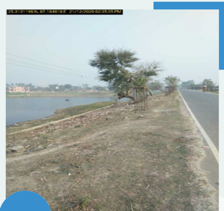
Road | BR_TINTANGA (PT-GOPALPUR) *_238978_013832_W2
